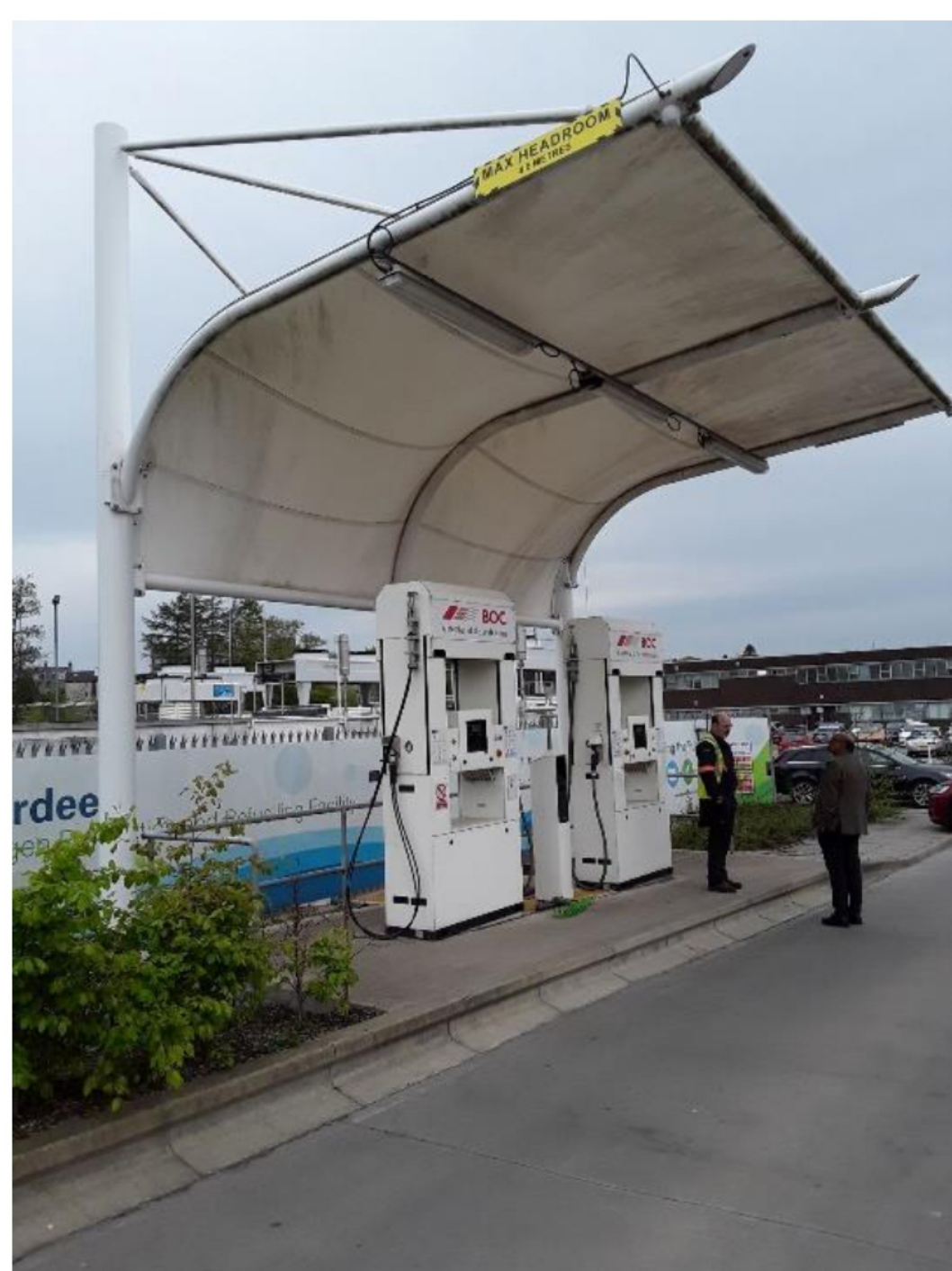
The Kittybrewster hydrogen refuelling station was opened in Aberdeen in 2015. It provides the local bus fleet, cars and vans with hydrogen fuel, which is produced in the electrolysers on site, as shown in the top two images. The design on the Argyll Hydrogen Hub will be similar to this.
