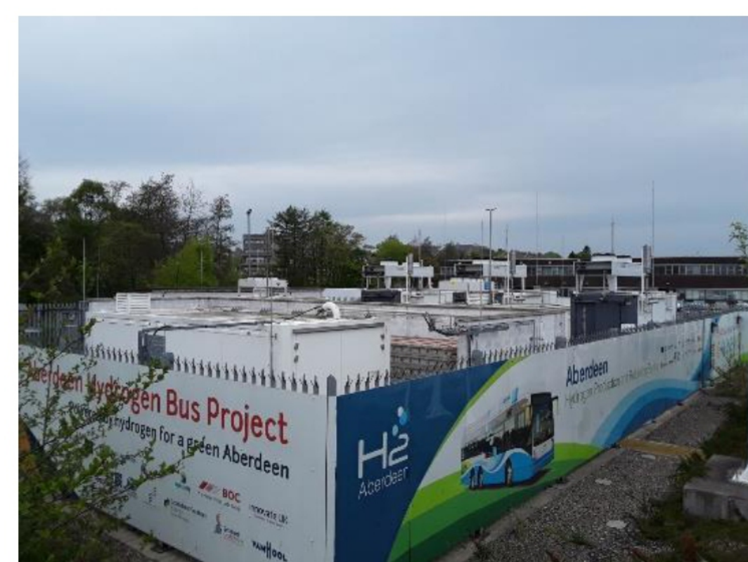
The Kittybrewster hydrogen refuelling station was opened in Aberdeen in 2015. It provides the local bus fleet, cars and vans with hydrogen fuel, which is produced in the electrolysers on site, as shown in the top two images. The design on the Argyll Hydrogen Hub will be similar to this.
